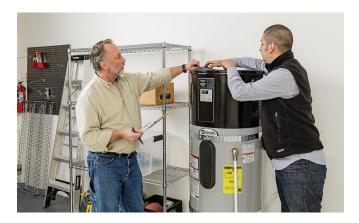
Fast replacements: The vast majority of installations (~80%) occur during "Normal Replacement" (NR) scenarios, meaning when the customer's WH has failed and they need a replacement as soon as possible. The main barriers to adoption for HPWH in these scenarios include the increased time required to replace a natural gas WH with a HPWH due to electrical upgrades, the lack of consumer knowledge, higher costs (for
